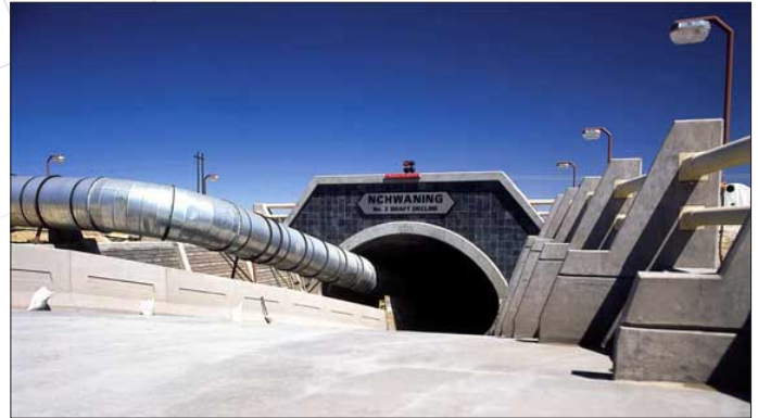
Nchwanging's 2,200 m inclined shaft
